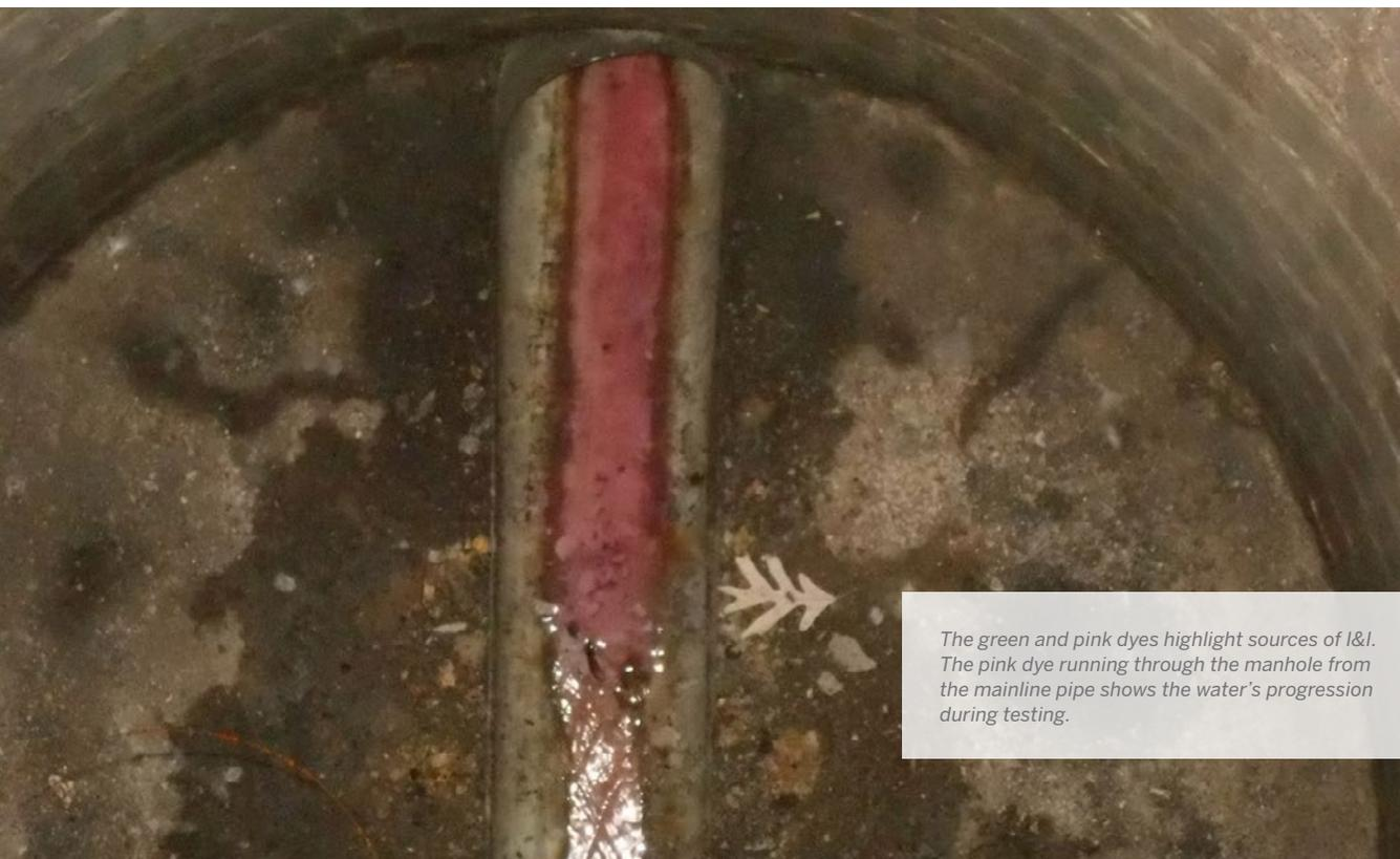
*The green and pink dyes highlight sources of I&I. The pink dye running through the manhole from the mainline pipe shows the water's progression during testing.*
